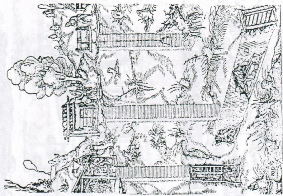
THREE VERTICAL TIMBERED SHAFTS, SERVED BY WINCHES (*Agricola*, f. 72).
